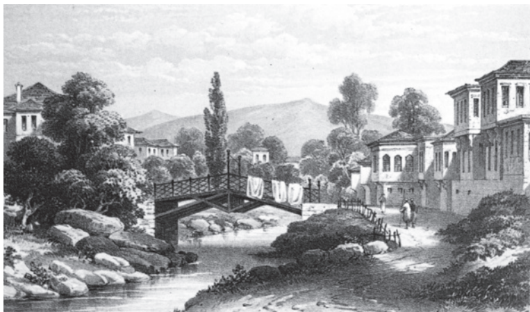
Fig. 3: Bridge on the Dragor – the first Western representation of Monastir/Bitola by Edward Lear in 1848. Source: Macedonia, 4000 years of Greek History and Civilization , Athens, 1892, p. 372.
